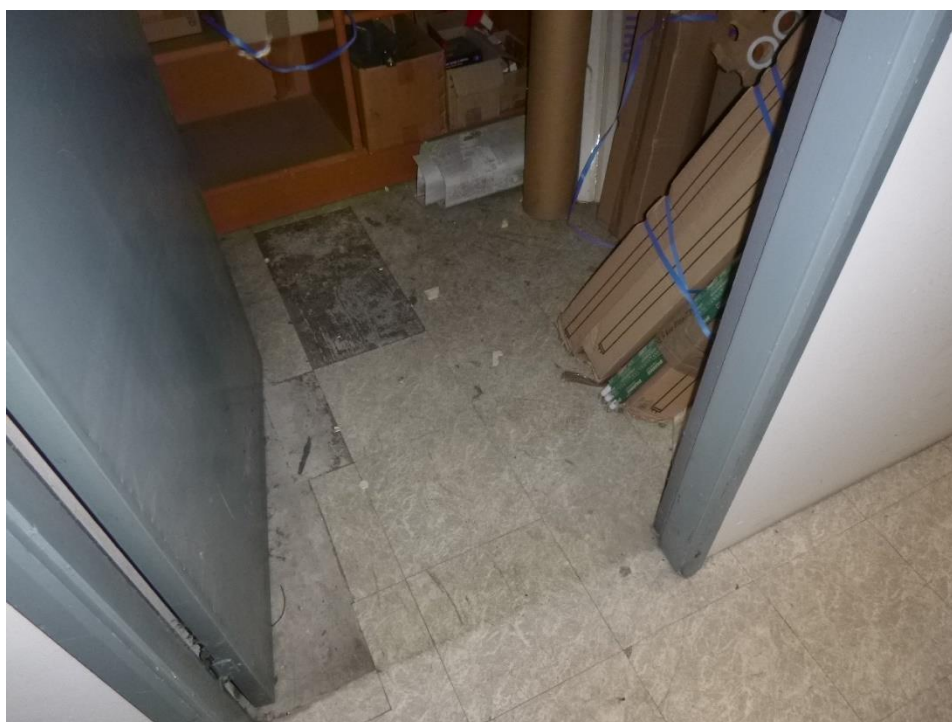
Plate 10 – Ground level, back of house areas, floor coverings, cream with grey speckles vinyl floor tiles. NAD Date: 09/03/2018
