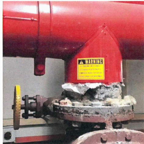
Photo 32. Level B2, Plant Room - Gasket
