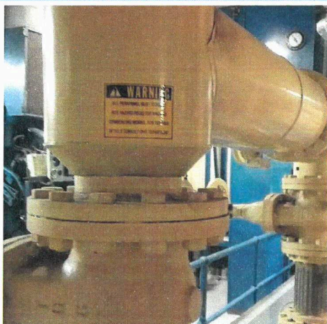
Photo 5. Level 23, Plant Room, Standby Pump 1, Hot Water Piping - Gasket
