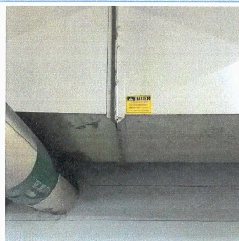
Photo 42. Level B1, Carpark, Ductwork - Mastic
