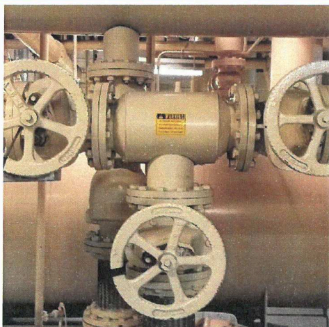
Photo 3. Level 23, Plant Room, Pump 1, Hot Water Piping, 3 Way Junction - Gasket
