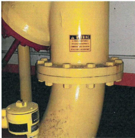
Photo 33. Level B2, Plant Room - Gasket
