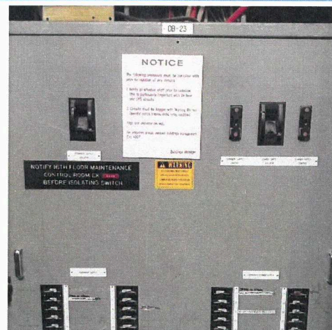
Photo 28. Level 23, Goods Lift, Electrical Switchboard - Bitumous Backing Board, Fuses
