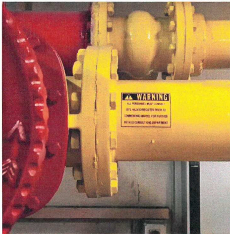
Photo 31. Level B2, Plant Room - Gasket
