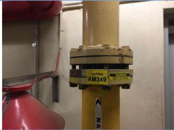
Photo 14. Interior, Ground Level - Plant room 2, adjacent to Data Room - Pipework - Gasket material - Assumed Asbestos containing material
