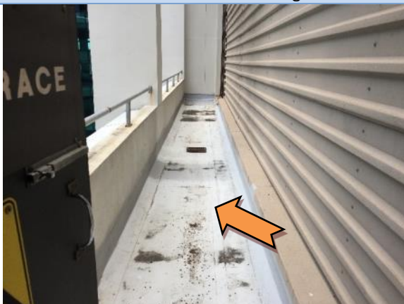
Photo 5. Exterior, Level 23 - Eastern Terrace accessed via Toilet Extraction Fan Room - Floor - Bituminous Membrane - Assumed Asbestos containing material
