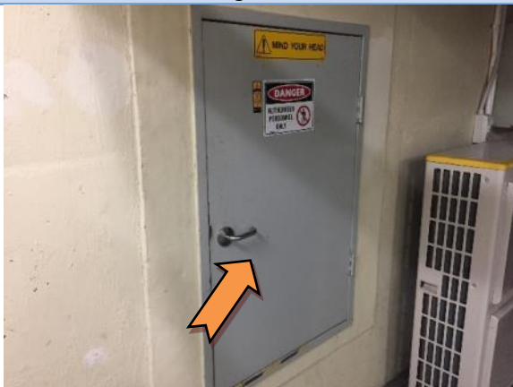
Photo 17. Interior, Ground Level - Plant Room 2, Duct Services Room - Door - Fire door core - Asbestos containing material - Removed May 2017
