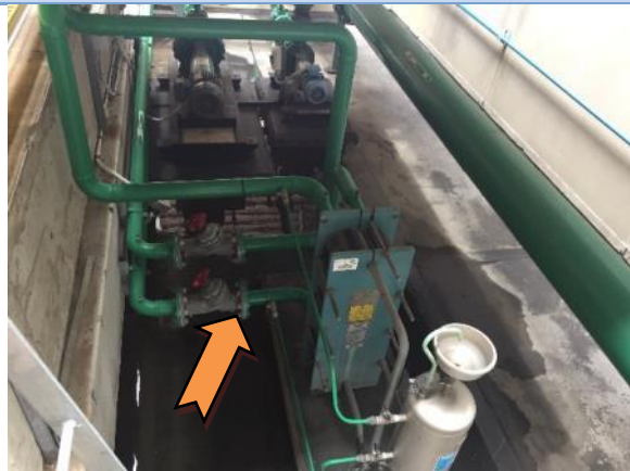
Photo 4. Exterior, Level 23 - Cooling tower condenser pump - Gasket - Gasket material - Asbestos containing material
