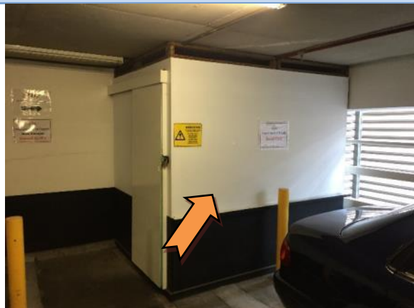
Photo 18. Interior, Level 2 - Department of Health & Ageing Store Room, Exterior - Walls - Fibre cement sheeting - Asbestos containing material
