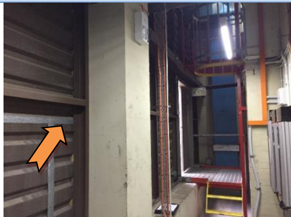
Photo 24. Interior, Level 23 - Plant Room, Northern Elevation - Wall - Galbestos - Assumed Asbestos containing material
