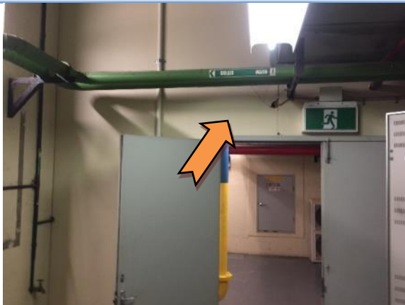
Photo 15. Interior, Ground Level - Plant room 2, Data Room - Partition Wall - Fibre cement sheeting - Assumed Asbestos containing material
