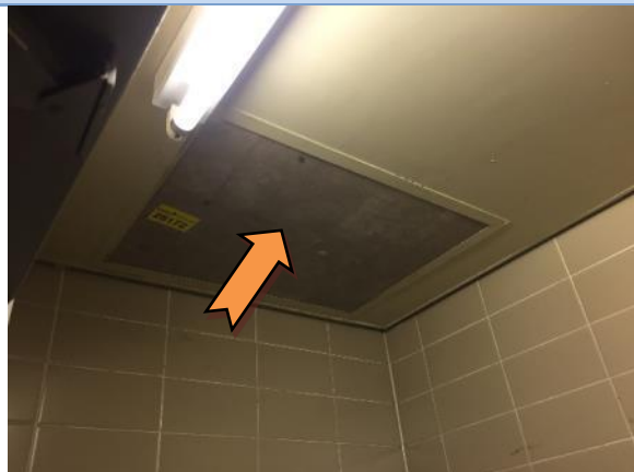
Photo 12. Interior, Ground Level - Plant Room 1, Washroom - Access hatch - Fibre cement sheet - Assumed Asbestos containing material - Removed May 2017
