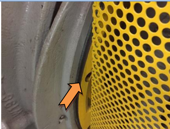
Photo 27. Interior, Level 24 - Lift Motor Room - Lift motor - Friction pads - Asbestos containing material
