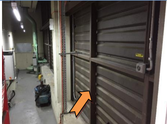
Photo 22. Interior, Level 23 - Fan Room, Southern Elevation - Wall - Galbestos - Assumed Asbestos containing material
