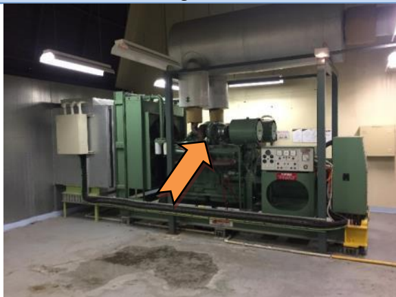
Photo 23. Interior, Level 23 - Generator Room - Gasket - Gasket material - Suspected Asbestos containing material
