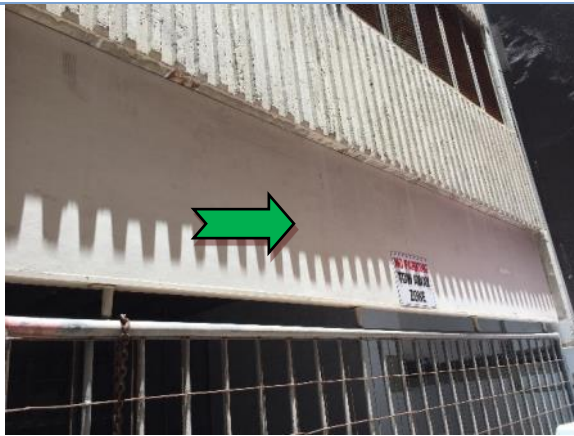
Photo 1. Exterior, Level 2 - Car Park, South-Eastern Corner, Above 'No Parking' bay - Infill panels - Fibre Cement Sheet - Non-asbestos containing material
