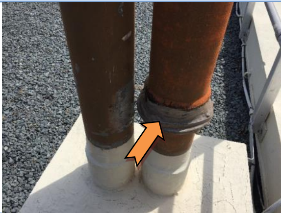
Photo 9. Exterior, Rooftop - Northern and Western Elevations - Flue - Mastic sealant - Assumed Asbestos containing material
