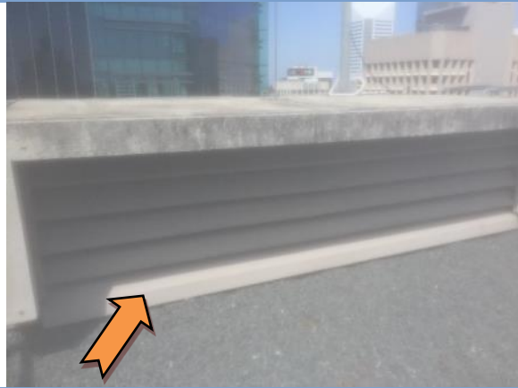
Photo 8. Exterior, Rooftop - Eastern Elevation, Fire Stairwell - Louvres - Galbestos - Assumed Asbestos containing material
