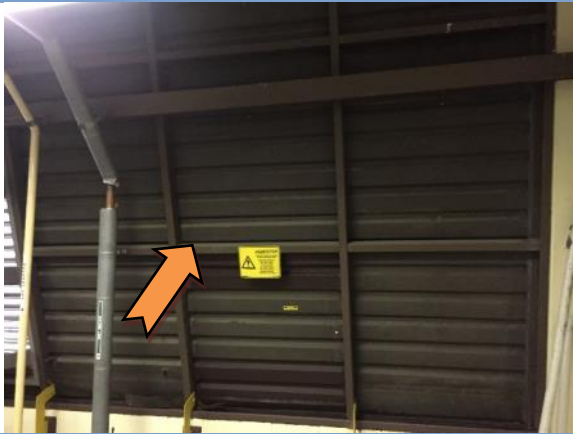
Photo 25. Interior, Level 23 - Plant Room, Southern Elevation - Louvres - Galbestos - Assumed Asbestos containing material
