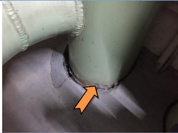
Photo 26. Interior, Level 23 - Fan room - Packer - Bituminous membrane - Asbestos containing material
