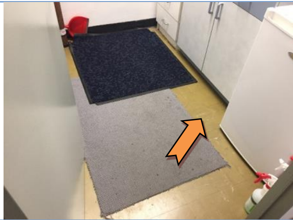
Photo 20. Interior, Level 22 - FM Office Kitchen - Floor coverings - brown (light) - Vinyl floor tiles - Assumed Asbestos containing material
