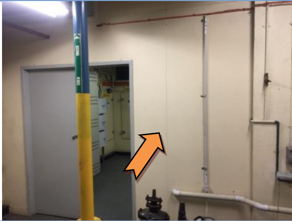
Photo 13. Interior, Ground Level - Plant room 2, adjacent to Data Room - Partition Wall - Fibre cement sheeting - Asbestos containing material
