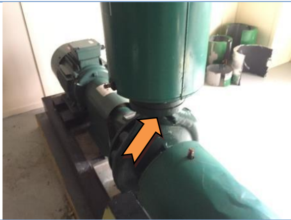
Photo 19. Interior, Level 22 - Chiller plant room - Pipe work - Gasket material - Asbestos containing material
