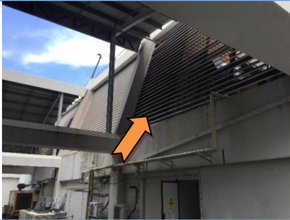
Photo 7. Exterior, Level 23 - Southern Elevation, Exterior Façade of Plant Room - Louvres - Galbestos - Assumed Asbestos containing material
