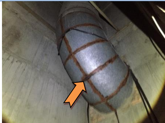
Photo 16. Interior, Ground Level - Plant Room 2, Duct Services Room - Duct - Mastic sealant - Assumed Asbestos containing material
