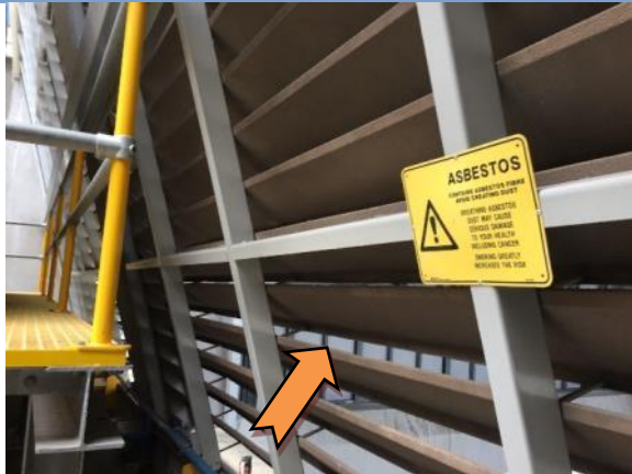
Photo 21. Interior, Level 23 - Cooling Tower Enclosure, Perimeter, All Elevations (Extends up to Level 24) - Walls - Galbestos - Assumed Asbestos containing material
