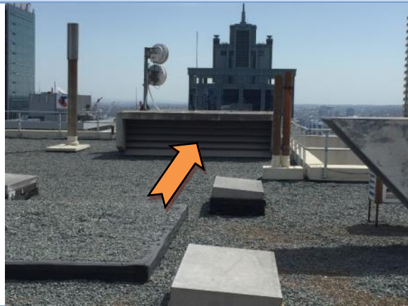
Photo 10. Exterior, Rooftop - Western Elevation, Fire Stairwell - Louvres - Galbestos - Assumed Asbestos containing material
