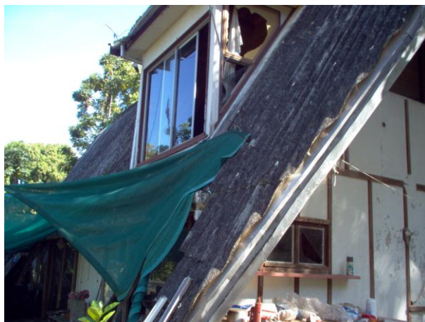
Example of ACM Roofing – Bonded
